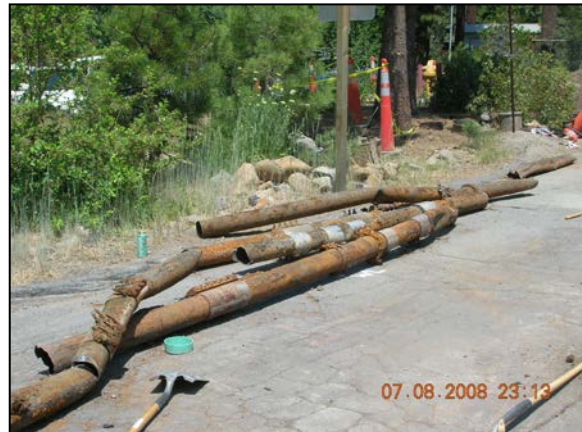
Aged Water Main Replacement (Photo courtesy of North Tahoe PUD)
